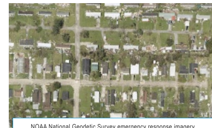
NOAA National Geodetic Survey emergency response imagery shows damage to buildings and homes in Houma, Louisiana, following Hurricane Ida.
