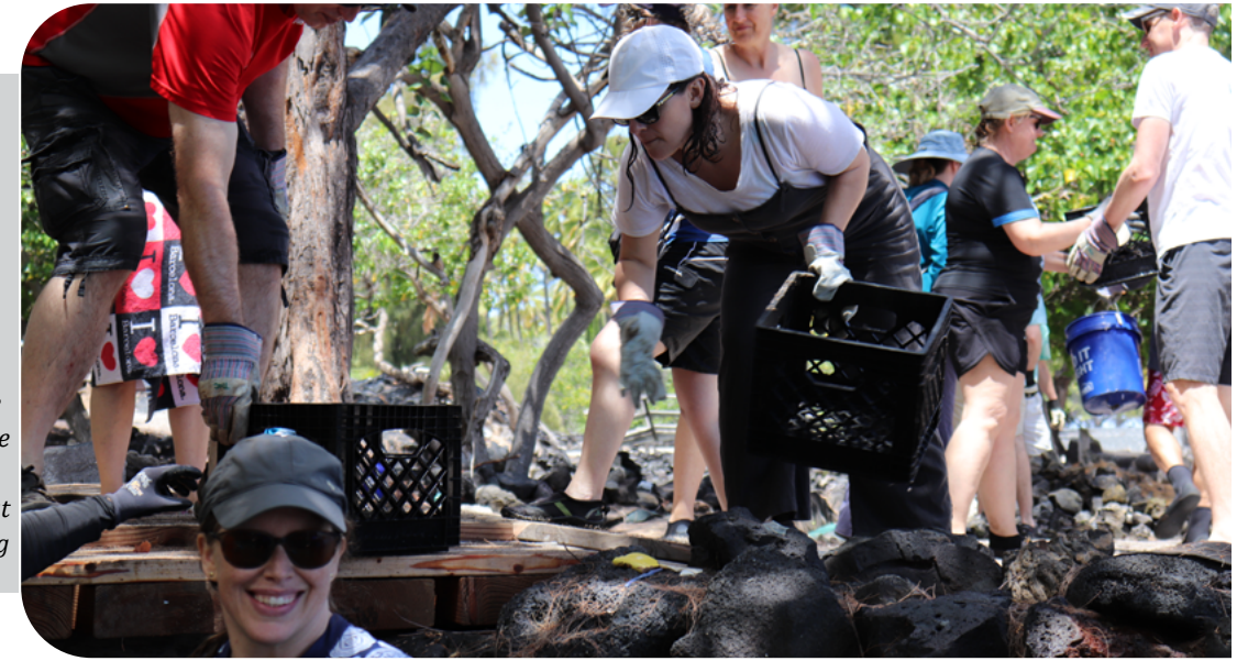
With NOAA's visit to West Hawai'i Habitat Focus Area at Kīholo Bay, workshop participants learned about traditional Hawaiian Fishponds as an ancient form of aquaculture helped gather rocks from the ponds. These rocks are used to rebuild and secure pond walls that were destroyed during a recent tsunami.
