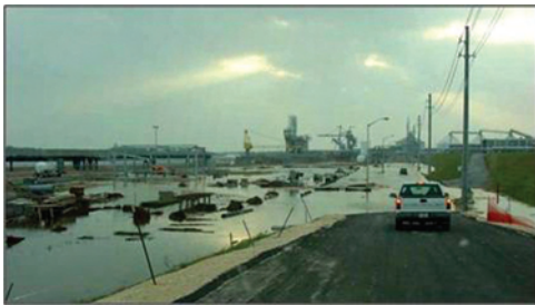
Surveying damage caused by storm surge from Hurricane Katrina
