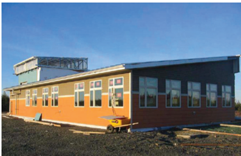
Construction of the Weather Service Office in Annette, Alaska
