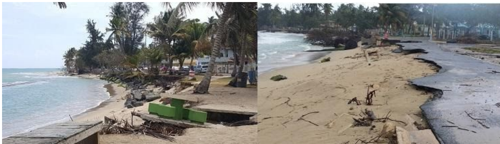
Figure 3. Photos showing coastal erosion problems, including damage to roads and recreation areas along the beach.
