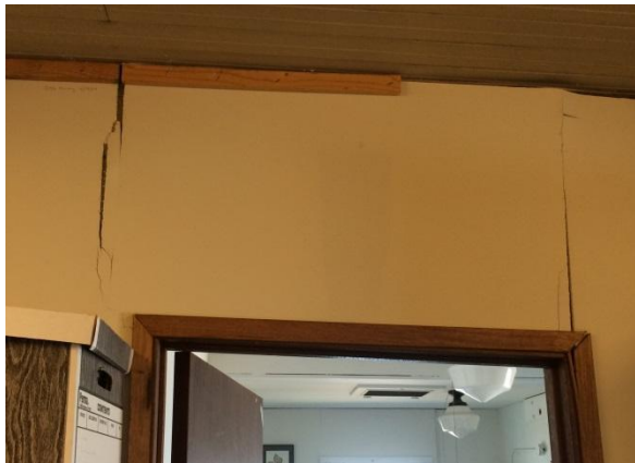
Fig. 2: Cracked walls from shifting foundation. Fig. 3: Jack network supporting the foundation.
