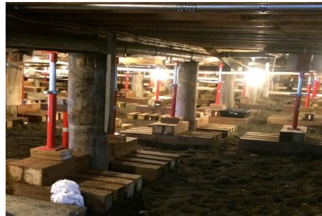
Fig. 2: Cracked walls from shifting foundation. Fig. 3: Jack network supporting the foundation.
