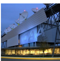
NOAA's Satellite Operations Facility in Suitland, Maryland. Photo credit: NOAA Photo Library, NOAA Satellites .
