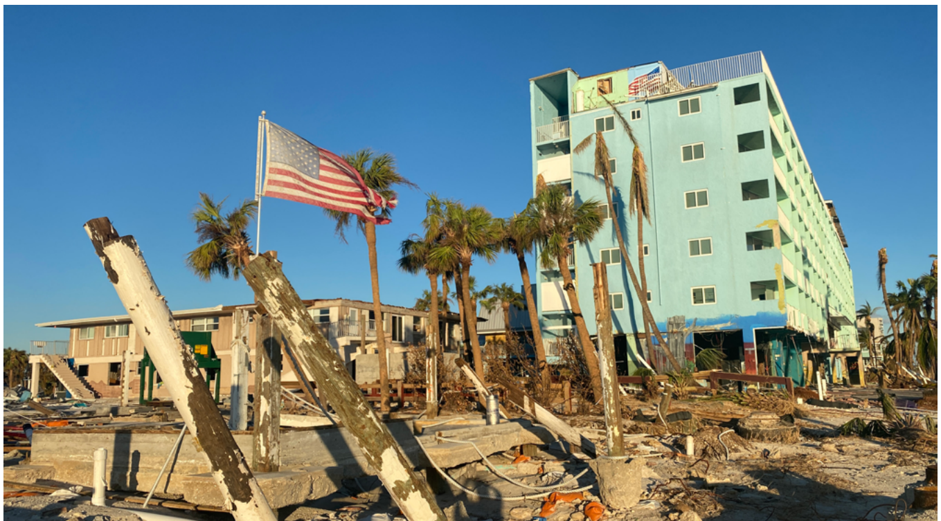
A flag blows in the wind among damage from Hurricane Ian in Fort Myers Beach, FL on Oct. 2, 2022. Credit: Jocelyn Augustino, Federal Emergency Management Administration
