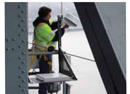
An employee from the Center for Operational Oceanographic Products and Services installs an air gap sensor which measures bridge clearance on the Verrazano-Narrows Bridge, New York. The sensor is part of the New York/New Jersey Physical Oceanographic Real-Time System. Information from the sensor is critical for under-bridge clearance, as ships continue to maximize channel depths and widths while, at the same time, push the bounds of bridge heights
