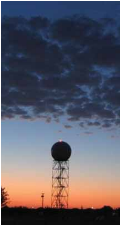
A Next Generation Weather Radar (NEXRAD). All NEXRAD systems are undergoing an upgrade to Dual Polarization capability to improve measurements, which are vital to increased accuracy and timeliness of warnings that protect life and property.
