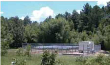
Wind profilers are specifically designed to measure vertical profiles of horizontal wind speed and direction. Data from this network are distributed in real-time to government and university atmospheric researchers, private meteorologists, the National Centers for Environmental Prediction, the Storm Prediction Center, all National Weather Service (NWS) Forecast Offices, and foreign agencies responsible for weather prediction.
