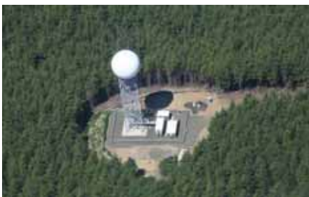
New NEXRAD Doppler installation in Kirkland, WA
