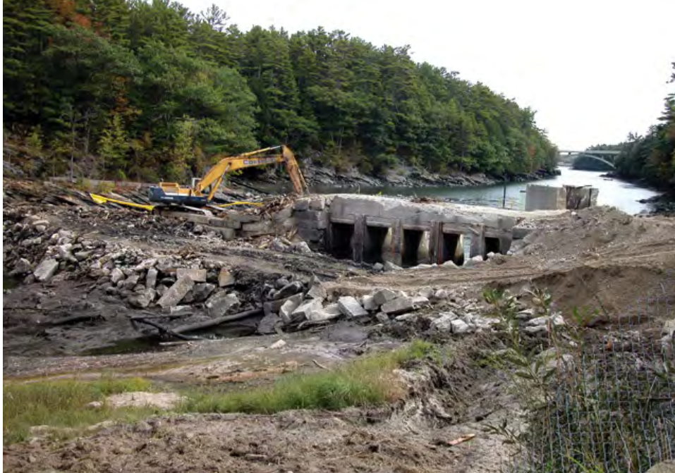
Removal of Smelt Hill dam under Open Rivers Initiative
