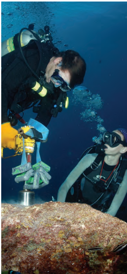
NOAA divers installing mooring buoy anchors using an underwater hydraulic drill at the Flower Garden Banks National Marine Sanctuary
