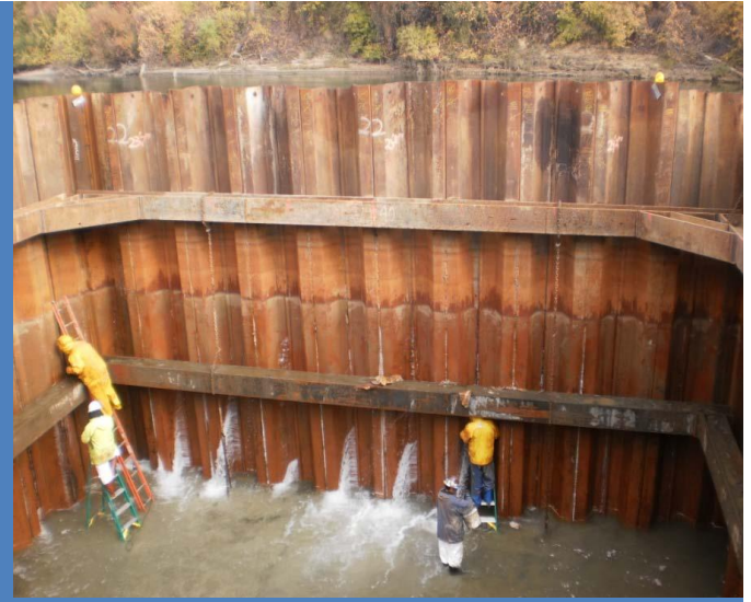
Coffer Dam at Yuba City
