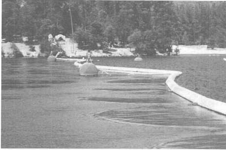
Figure 15. - Photograph of the Carr tailrace curtain billowing upstream, which was caused by a large differential density load. Flow from Carr powerplant moves from left to right.
