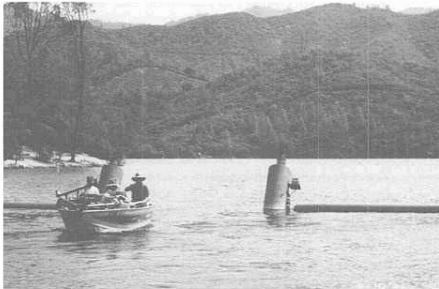
Figure 6. - Photograph of the 16-ft-wide, 6-ft deep boat passage in the Carr Powerplant tailrace curtain.
