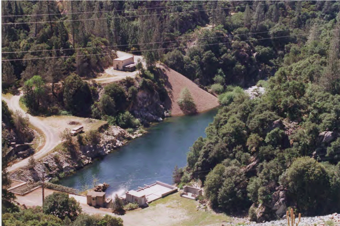
Figure 4. USBR/WSRCD gravel augmentation site directly downstream of Whiskeytown Dam in Lower Clear Creek. This method offers convenience and efficiency, but often requires many years before a spill event distributes gravels downstream to areas that will benefit salmonids.
