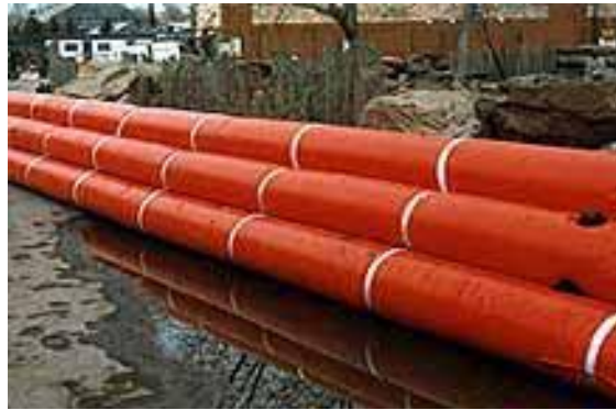
Figure 29. Example of bladders for temporary weir.
