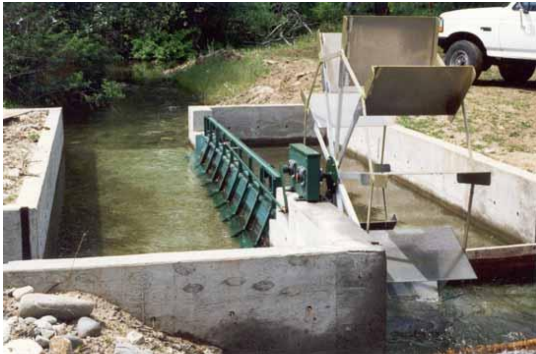
Figure 22. Lower Etna Creek diversion screen, Siskiyou County.
