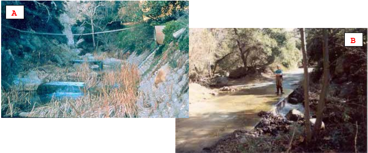
Figure 6. Southern California stream urbanization: Concrete channelization (A) and Ford crossing migration barriers (B).
