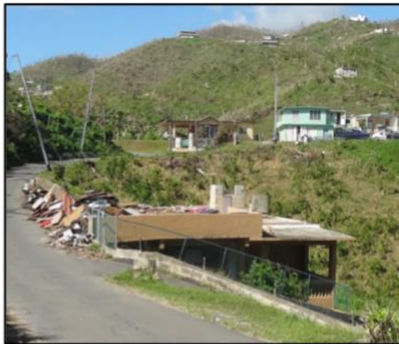
Figure 1. Damage associated with topographic wind speed up
