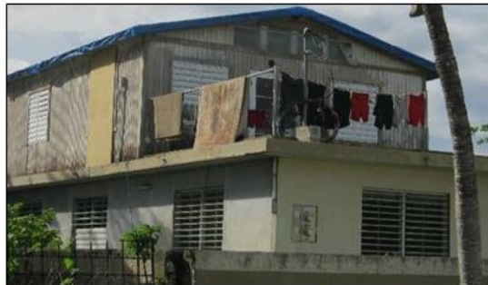
2 Story House: 1 st Floor CMU Walls with Concrete 2 nd Floor and Wood Walls at 2 nd Floor with Wood Roof
