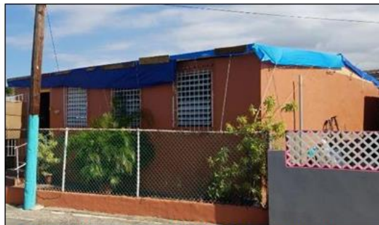
1 Story House: CMU Walls with Wood Roof
