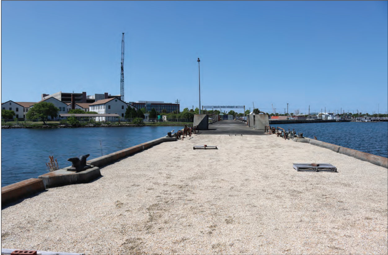
Figure 4.1 SHPO Site No. 8422, Pier Romeo, facing southwest.
