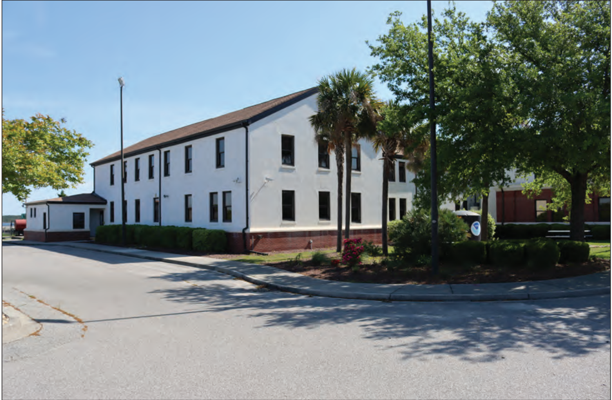
Figure 4.7 SHPO Site No. 8423, RTC-1, southwest oblique facing northeast.
