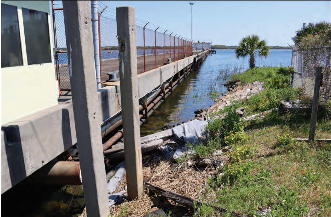
Figure 4.3 SHPO Site No. 8422, Pier Romeo, south elevation, facing northeast.
