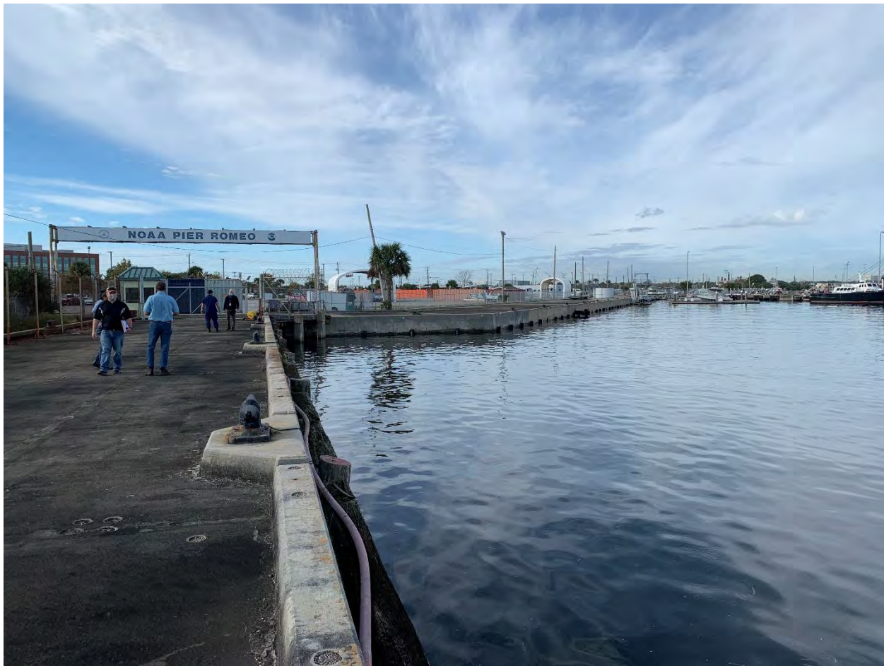
Photo 2: View of Pier Romeo facing southwest. Photo taken May 2021.
