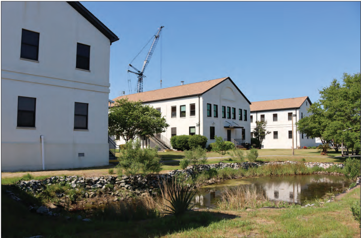
Figure 4.8 SHPO Site No. 8423, RTC-1, rear elevation, facing southwest.
