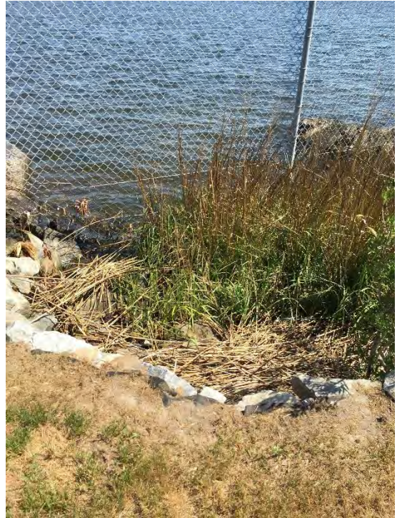
Photo 3: Photo of rip rap at shoreline adjacent to Pier Romeo
