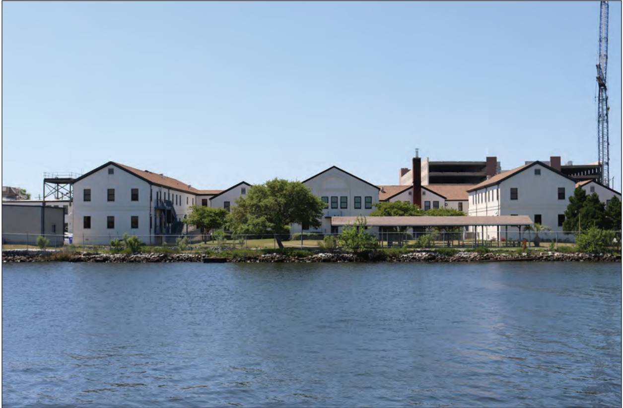
Figure 4.6 SHPO Site No. 8423, RTC-1, rear elevation, facing south.
