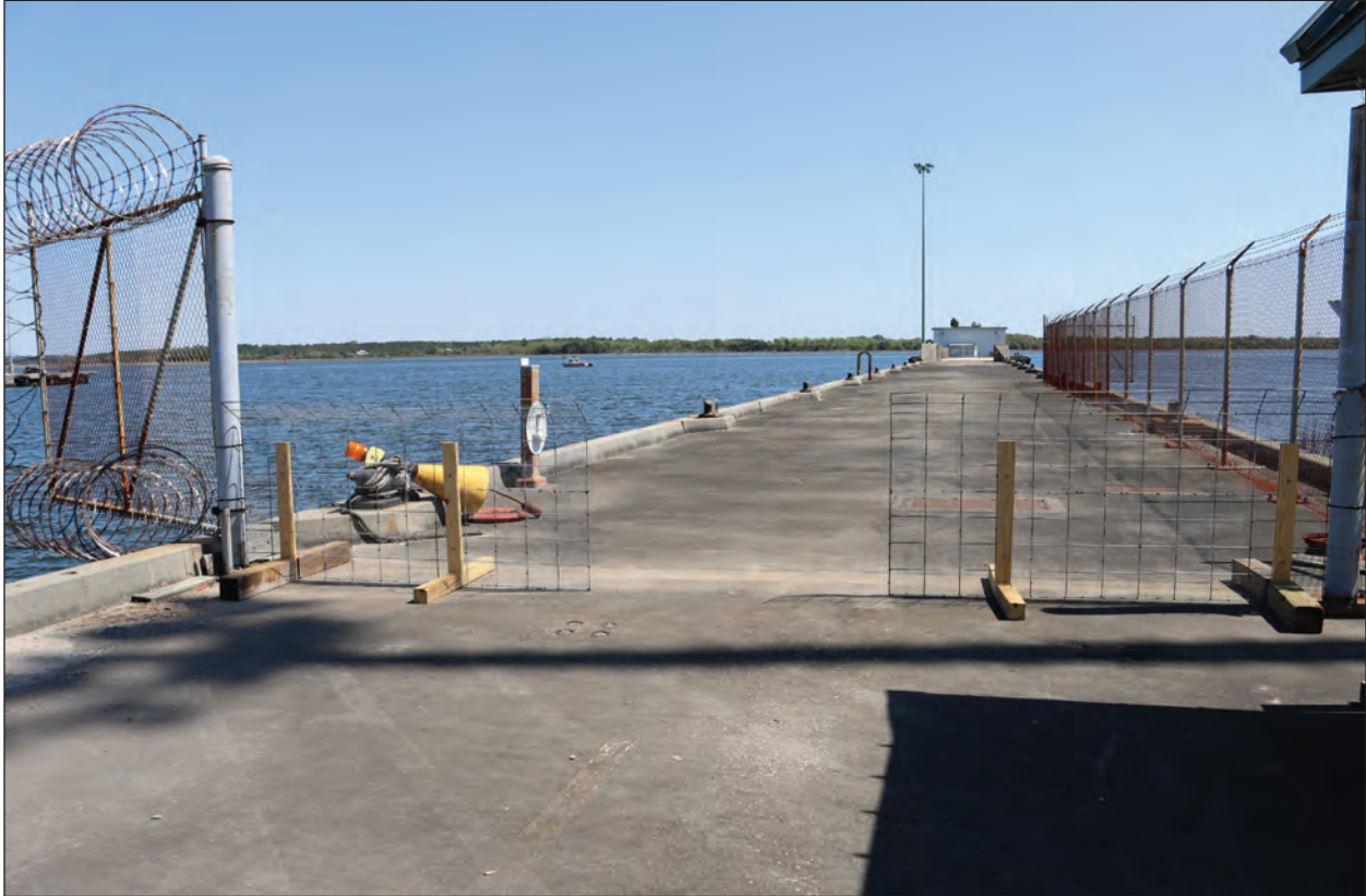
Figure 4.4 SHPO Site No. 8422, Pier Romeo, facing northeast from Sentry house.
