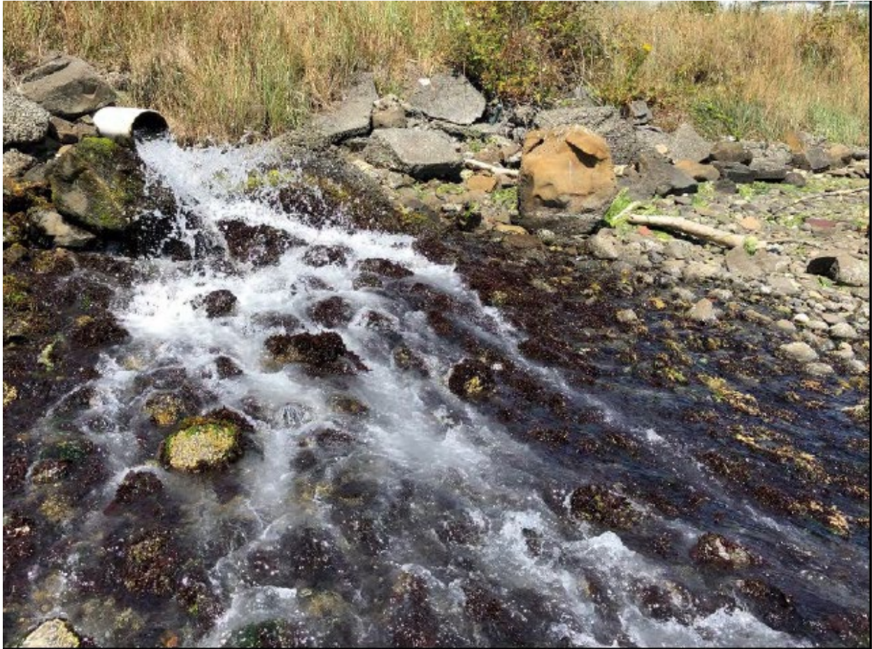
Figure 4.5-2 Existing Discharge at Main Outfall during low tide conditions
