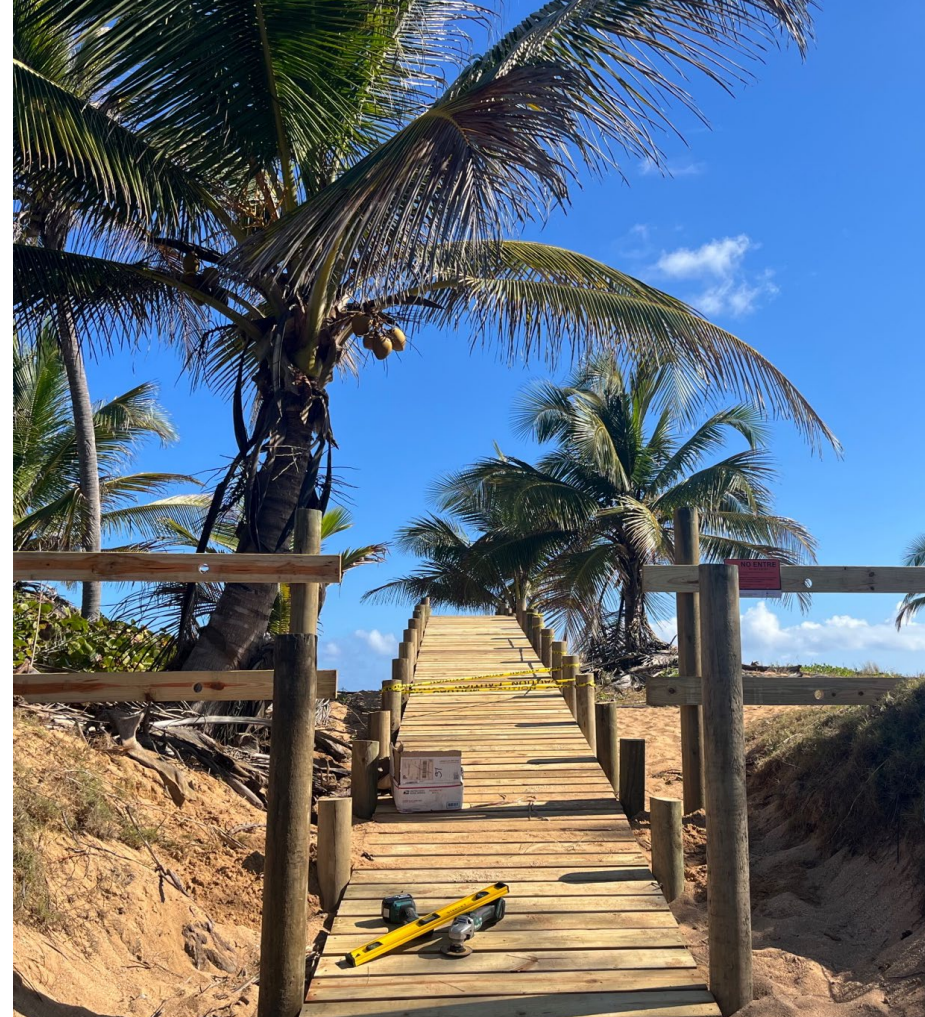
Playa Tocones, Loiza. Installation of 60 ft of exclusion fences. March 08, 2024.
