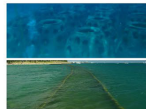
2 PHOTO 2 - Underwater Breakwater
