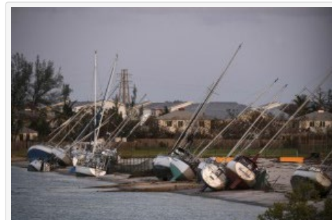
Hurricane Irma Damage in Florida Keys
