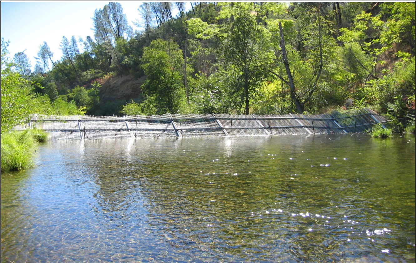
FIGURE 2.—The Clear Creek temporary picket weir installed at river mile 8.09 during September and October, 2003 and 2004, to spatially separate spawning spring-run and fall-run Chinook .
