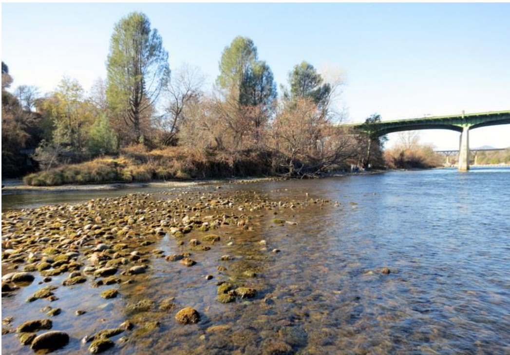
Figure A-9. Looking upstream (river left) across the river to Site 3.
