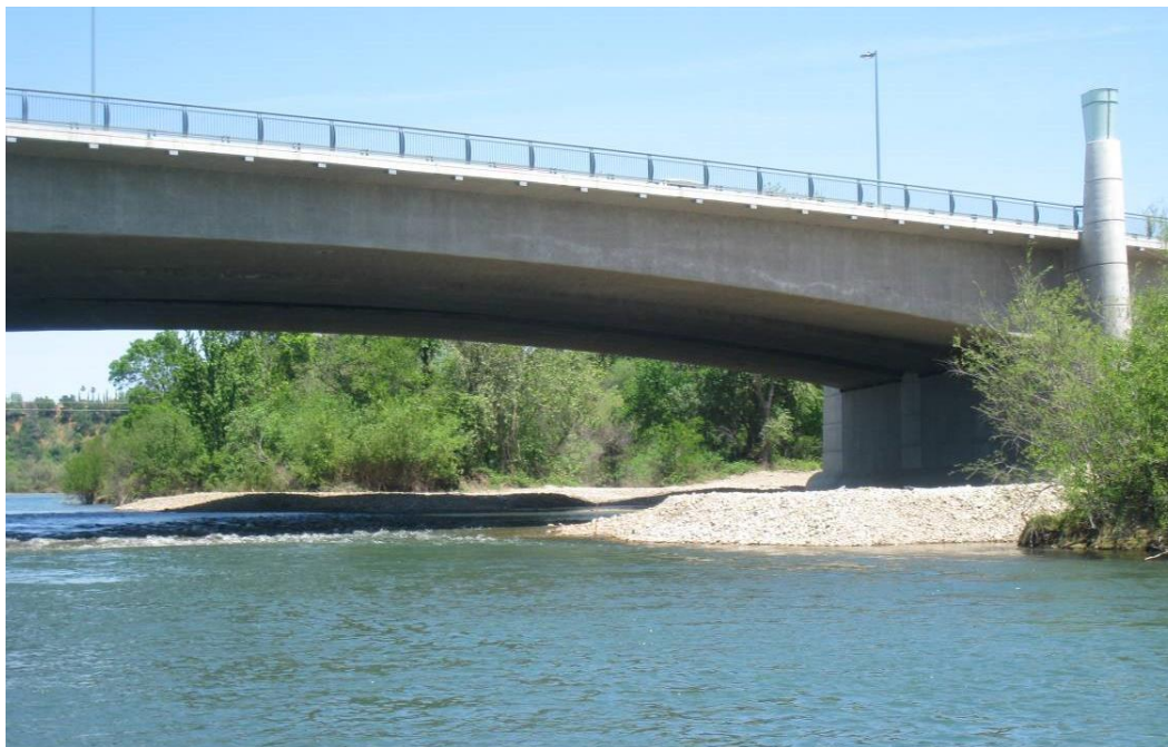
Figure A-14. Cypress Avenue Bridge North (Site 6) looking upstream across the river at the southeastern end of site.
