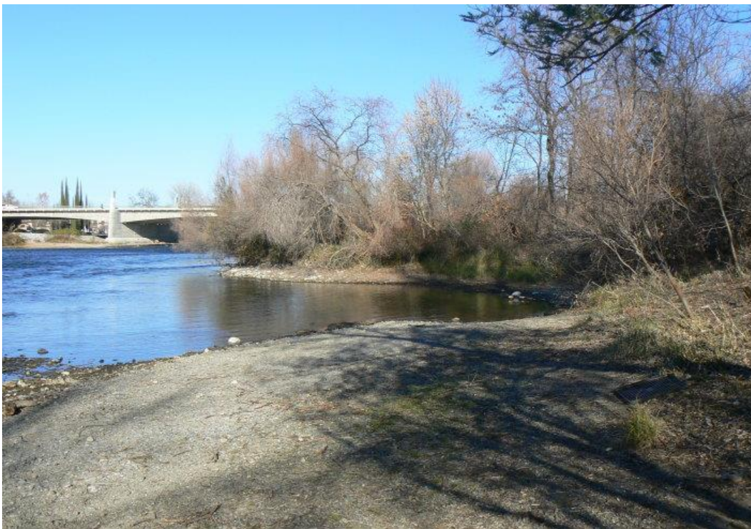
Figure A-17. Cypress Ave Bridge South (Site 7) on river right.
