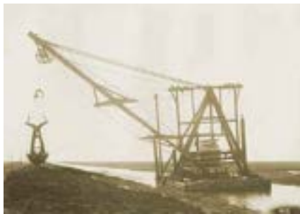
Figure 1.15. Clam-shell dredge building levees. The clam-shell dredge, Vulcan, is shown building the height of an artificial levee along an unknown waterway. After initial reclamation efforts, where levees were built primarily by Chinese laborers, dredges were used to build higher levees to keep out the tides and floods. (McCurry Foto Co. ca. 1910, courtesy of the California History Room, California State Library, Sacramento)
