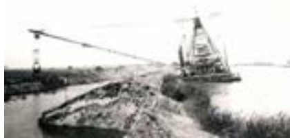
Figure 4.14. Dredge building levee showing side-ditch. This early 1900s photograph shows a side-draft clamshell dredge working on a levee, drawing material from a ditch. Over the past century, many of these ditches have become a part of the main channel. (Covello ca. 1900, courtesy of Bank of Stockton Historical Photograph Collection)
