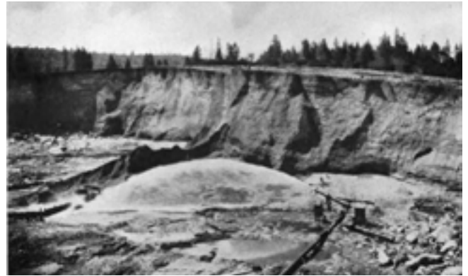
Figure 1.13. Hydraulic mining. The caption of this photograph, which is shown as Plate I of Grove Karl Gilbert's treatise on hydraulic mining debris (1917), reads: "A hydraulic gold mine. The water is conveyed by pipe, under a head of several hundred feet, and delivered through a nozzle that can be turned in any direction. The jet washes the auriferous earth from the cliff and thence to a sluice, seen at the left. The sluice is several hundred feet long and contains pockets of mercury by which the gold is caught." (photo by Gilbert 1908, from Gilbert 1917)
