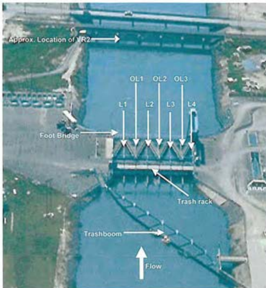
Figure 20. Acoustic tag range testing positions within the SFPF louvers. The acoustic tag (VEMCO, model V8SC) was lowered into the water at the trashboom, at the trash rack, inside the louver bays (L1, L2, L3, L4), outside the louver bays (OL1, OL2, OL3), and at the foot bridge.
