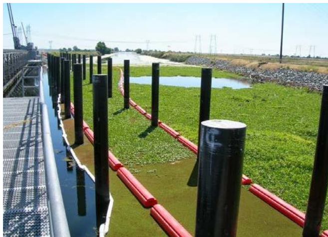
Figure 8. View upstream (east) of aquatic weeds in Rock Slough (Reclamation 2016).
