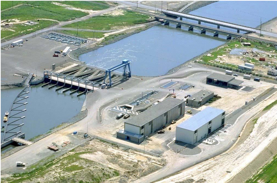
Figure 1 -Aerial view of the SDFPF including the Primary Louvers arranged in a Vee configuration
