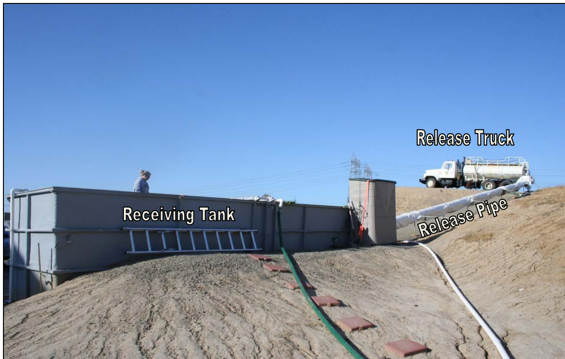
Figure 5- Mock release site constructed at the SDFPF compound.
