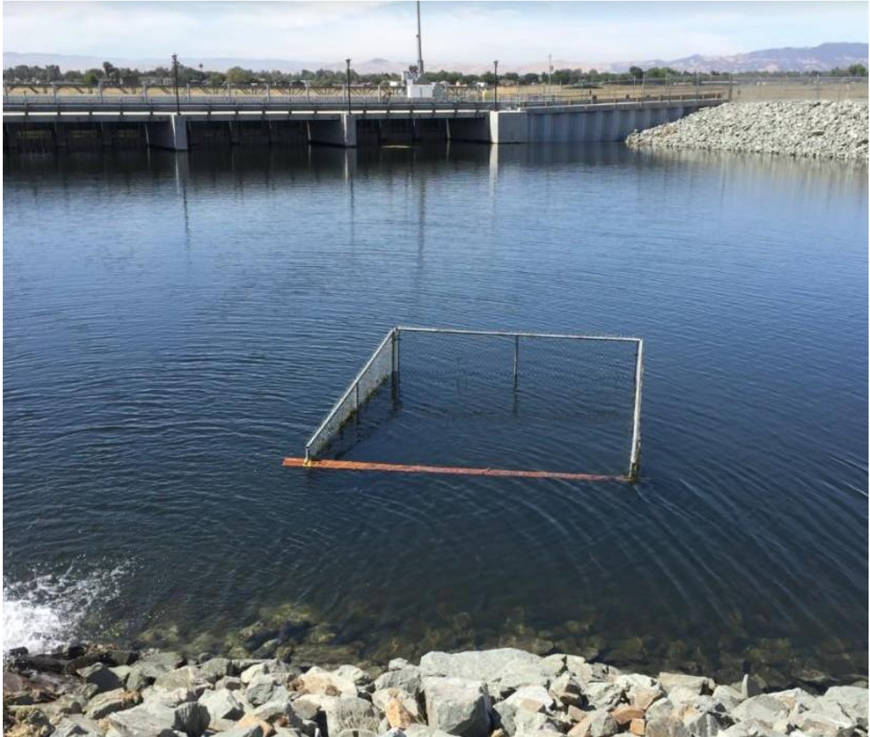
Figure 13 Photograph of Chain Link Fence Surrounding Ranchers' Intake
