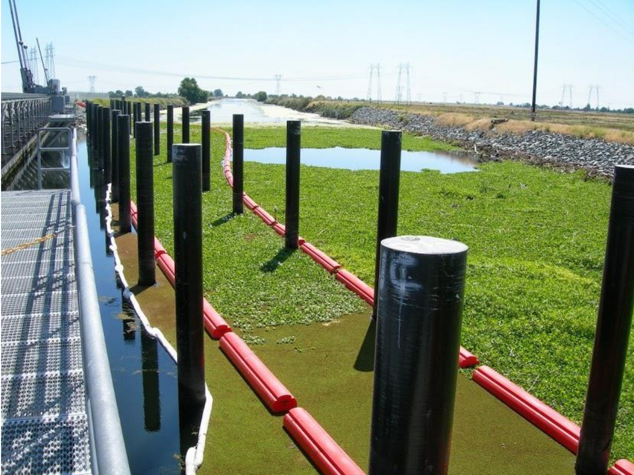
Figure 15 Aquatic Weeds at the RSFS Facility
