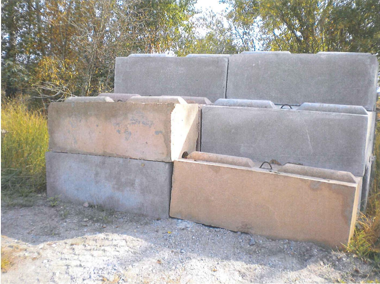
Figure 11 Photograph of the Ecology Block used to Anchor the Relocated Log Boom
