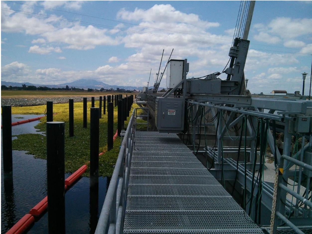
Figure 5 Existing Safety Deck on the Northeast side of the RSFS
