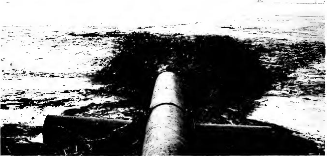
Figure 7. Dredged material discharged from a pipeline dredge. Photo courtesy of FWS, Ecological Services, Lafayette, Louisiana.
