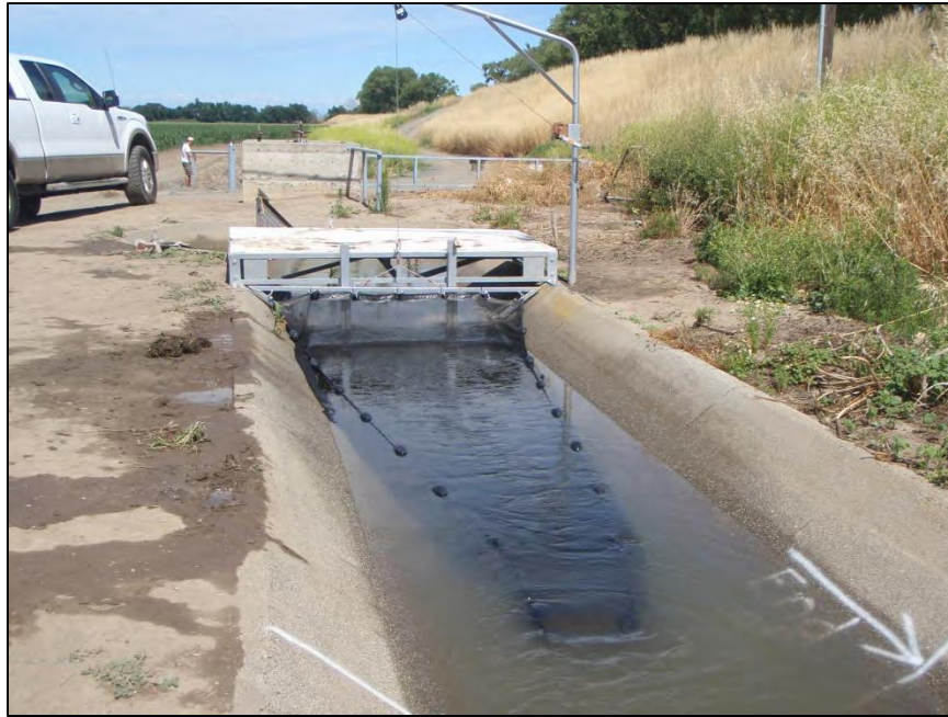
Figure 6. Fyke apparatus and sampling platform used for fish entrainment sampling in the South Steiner concrete canal.
