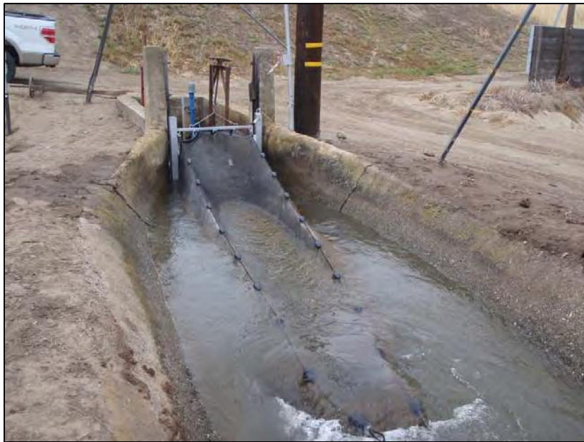
Figure 13. The fyke net and associated apparatus used to sample for fish entrainment in the Cranmore trapezoidal concrete canal.
