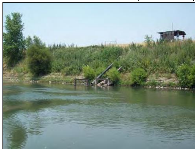
Appendix Figure 23. The South Steiner pump station intakes looking in a downstream direction.
