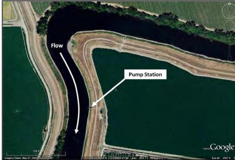
Appendix Figure 29. Location of the Oji pump station on the Sacramento River.
