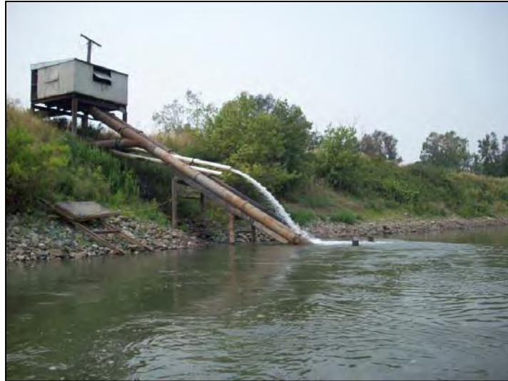
Figure 118. An example of excess flow at an unscreened diversion being diverted back into the Sacramento River.
