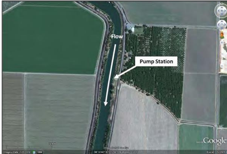
Appendix Figure 64. Location of the Tisdale pump station on the Sacramento River.
