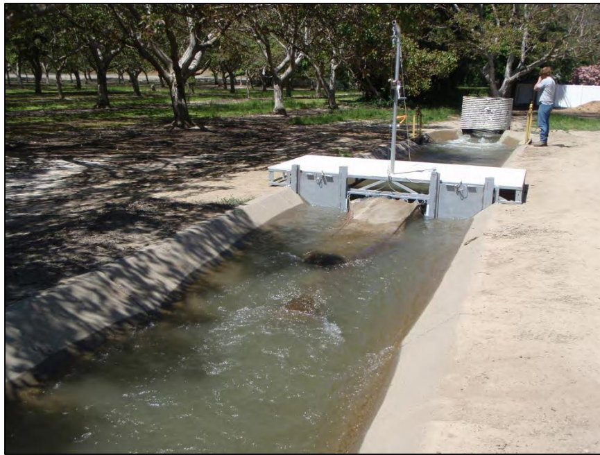
Figure 10. The fyke net, sampling platform, and associated apparatus used to sample for fish entrapment in the Alamo trapezoidal concrete canal.
