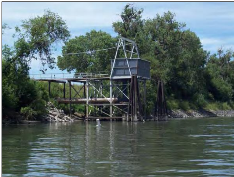
Appendix Figure 58. The Townsite pump intakes looking in an upstream direction.
