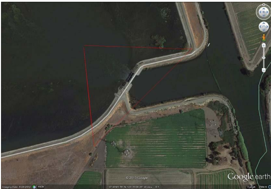
Figure 31: Restricted Access in the vicinity of Radial Gates
