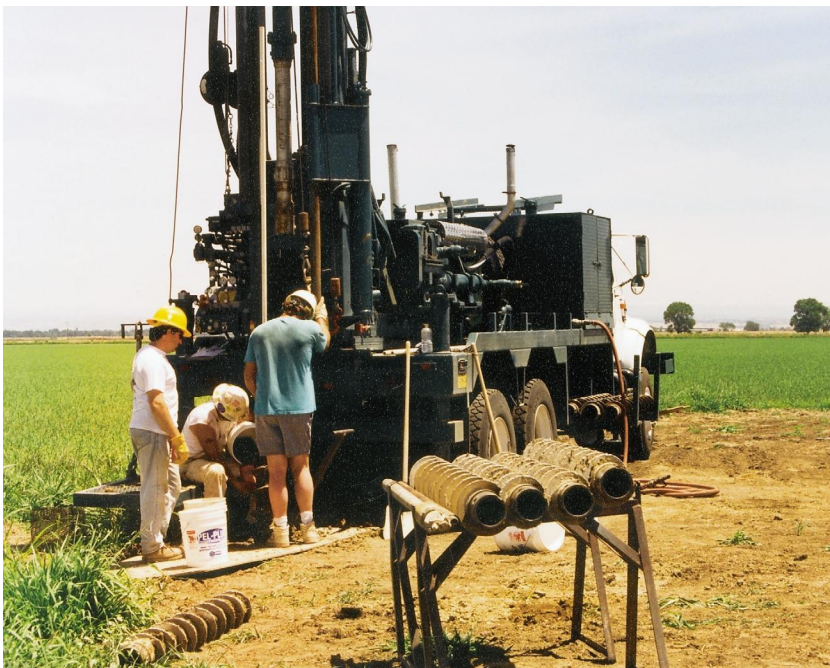
Figure 20. Drilling and installing a new monitoring well in the rice-growing region of the Sacramento Valley.
