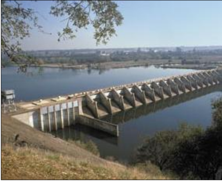
Nimbus Dam and Lake Natoma.
