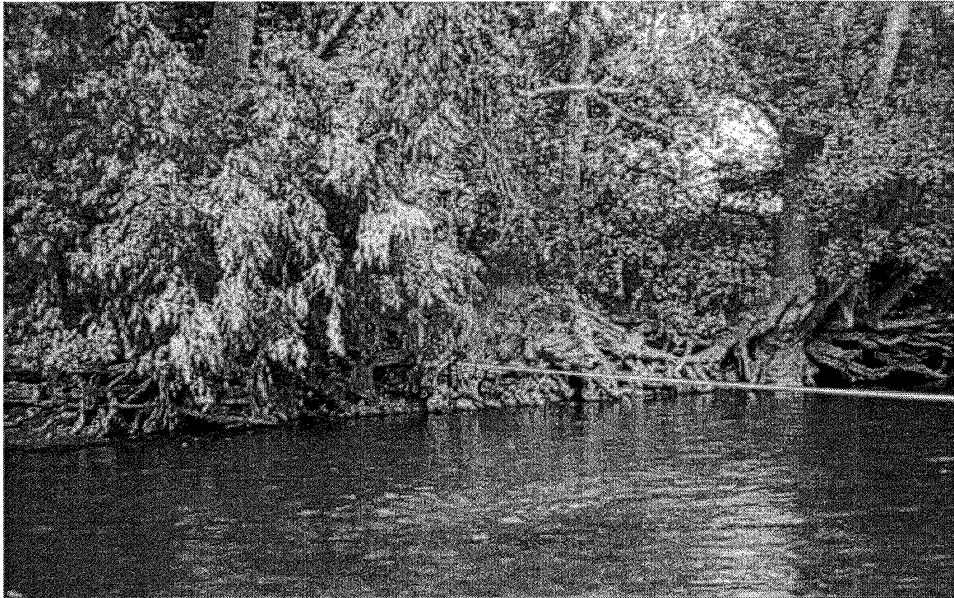
Figure 5.5: Root Crown Exposure at R78, Stanislaus River. (RM 40: 375cfs). Note the vegetation encroachment and extent of root wad exposure at this site, indicating channel incision and erosional processes (Photo, K. Schneider, 10/27/99).
