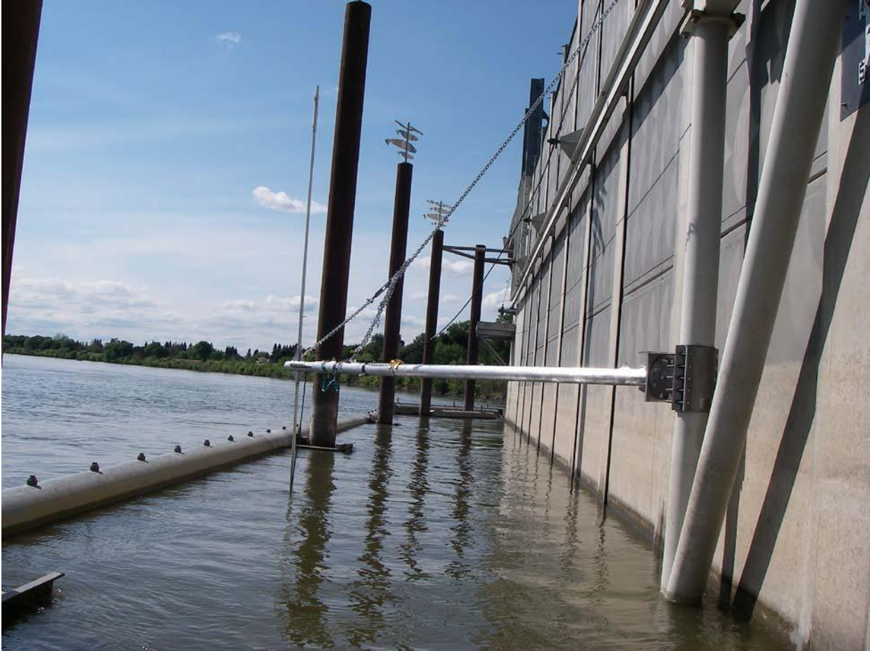
Figure 5. DIDSON/ARIS Pole Mount Attached to Fish Screen Cleaner Assembly
