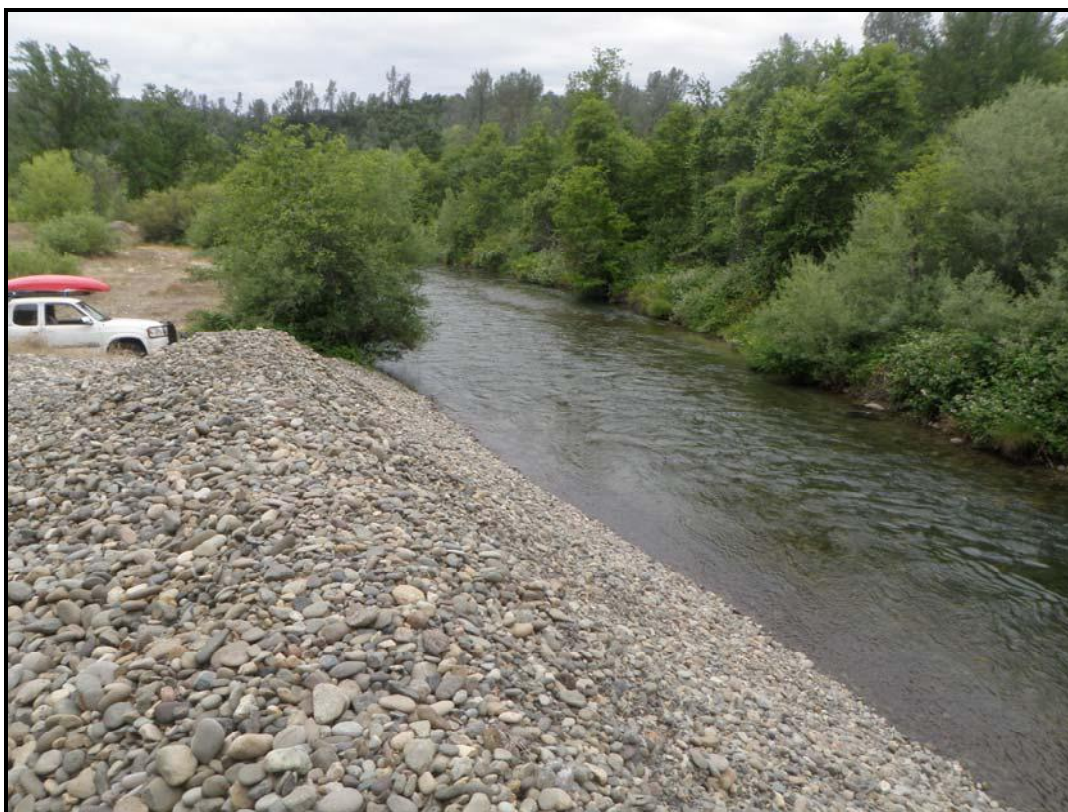
Figure 15. Downstream view of the Clear Creek Road gravel injection, June 2011.
