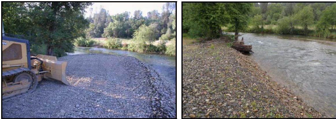
Figure 19. Downstream views of the 2010 injection efforts above Phase 3A pre and post-winter high flows. Note the exposed claypan in the post-winter photo.
